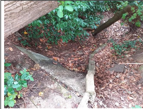
Fig 6: Dry Spillway at the eastern end of the lake
